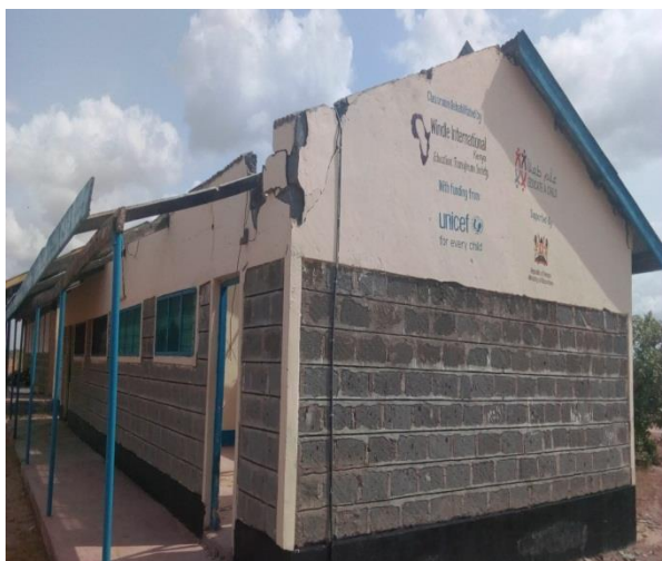
The damaged roof of Kumahumato Primary School standard 7 & 8 classroom block
