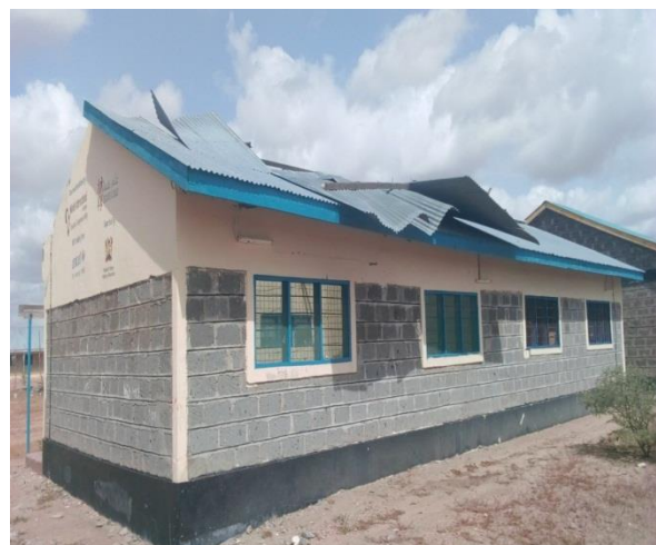
The damaged roof of Kumahumato Primary School standard 7 & 8 classroom block
